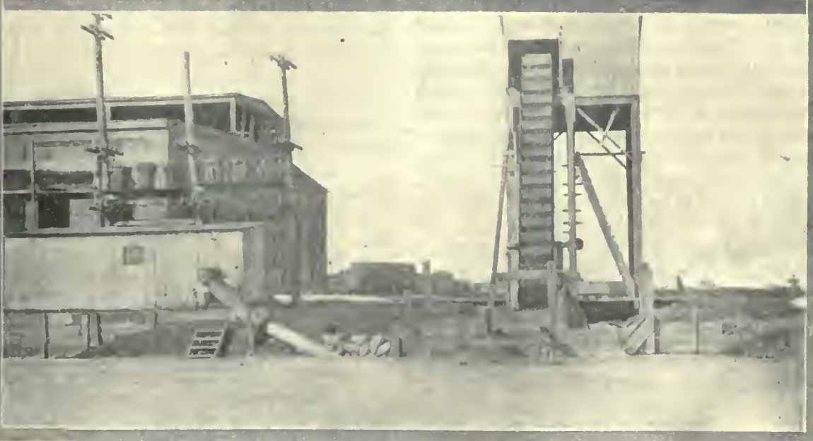
CARS OF COAL ARE DUMPED THROUGH THE TRESTLE SHOWN IN THE UPPER PICTURE AND FLUSHED INTO THE POND, BEING DISTRIBUTED TO ANY POINT BY MEANS OF THE DELIVERY PIPE SHOWN IN THE MIDDLE, AND LOADED OUT BY MEANS OF THE ELEVATOR SHOWN IN THE LOWER PICTURE.
